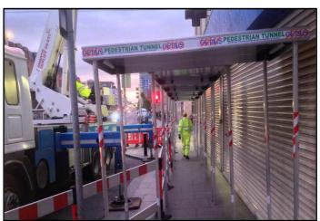
All four aluminium telescopic legs have a patented device within its design, this allows them to quickly and accurately unfold and lock into position. The Pedestrian Tunnel is then ready to use and help protect people from falling objects.
