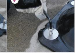
Position product centering the four holes. The fixing screws should drop down until they Remember to make sure the front of the bollard reach the threaded part of the Anchor. Make faces oncoming traffic. Place the large washers sure all four bolts are engaged in the shield over the button head screws and place through thread by 2 or three turns then proceed to the nylon inserts and into the Anchor. tighten all four bolts to torque setting 27.
