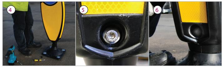
Place the new bollard top over the screw thread Place the M8 washer over the replacement M8 Using the Allen key, tighten the M8 x 120mm and rotate until screwed down to its full extent. x 120mm long Socket head cap screw. Ensure long Socket head cap screw to a torque of min (Lubricating the screw threads with a silicone the holes correctly align and push the socket 4 Nm max 4.5 Nm. Push in the replacement polish or a little grease may make this easier). head cap screw into the assembly.
