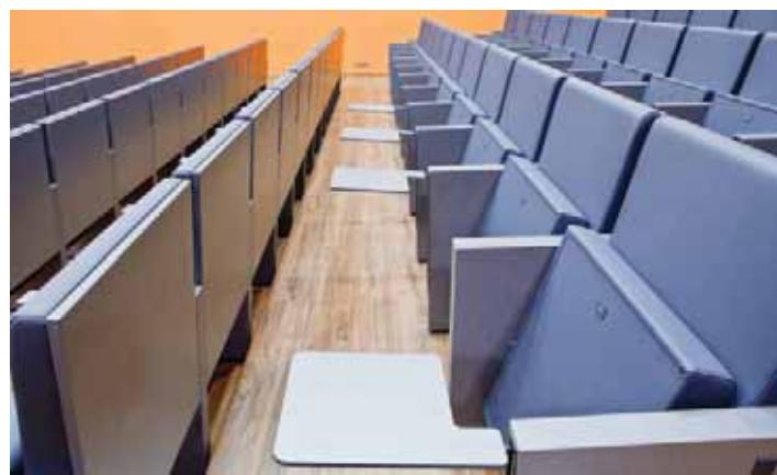
**Detail of micro-perforated seat base and retractable tablet.**
