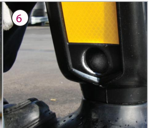
Place the new bollard top over the screw thread and rotate until screwed down to its full extent. (Lubricating the screw threads with a silicone polish or a little grease may make this easier).
