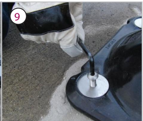
8 The fixing screws should drop down until they anchor shields so the thread end is just past the Remember to make sure the front of the bollard reach the threaded part of the shield. Make sure all four bolts are engaged in the shield thread by top of the anchor is flush with ground level. Tap over the button head screws and place through 2 or three turns then proceed to tighten all four bolts to torque setting 27.
