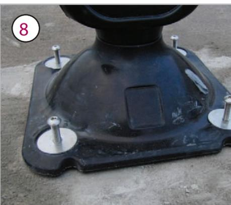
8 Position product centering the four holes. Remember to make sure the front of the bollard reach the threaded part of the Anchor. Make faces oncoming traffic.
