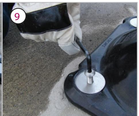
9 The fixing screws should drop down until they sure all four bolts are engaged in the shield over the button head screws and place through thread by 2 or three turns then proceed to tighten all four bolts to torque setting 27.
