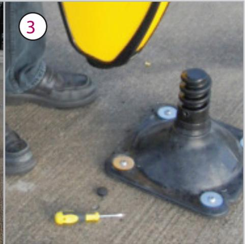
Using a small screwdriver remove the plastic cap on the right hand side of the bollard (right hand side when facing the front of the bollard).
