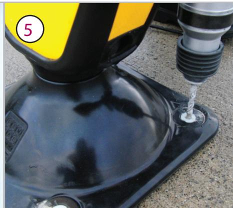
5 Using the product base (with nylon spacers fitted) as a jig, drill 10mm diameter holes to a depth of approximately 5-10mm, to mark hole centres.
