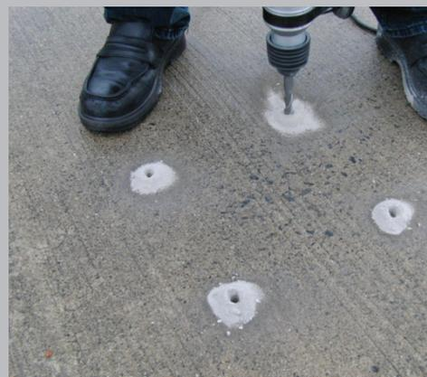
10 mm masonry drill bit
