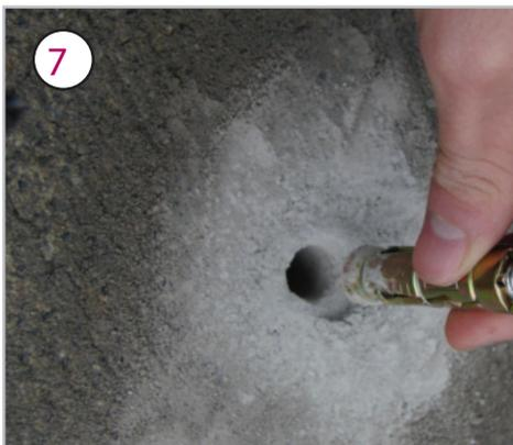
7 Screw the 100mm button head screws into the Position product centering the four holes. Remember to make sure the front of the bollard reach the threaded part of the shield. Make sure all four bolts are engaged in the shield thread by top of the anchor is flush with ground level. Tap over the button head screws and place through 2 or three turns then proceed to tighten all four bolts to torque setting 27.
